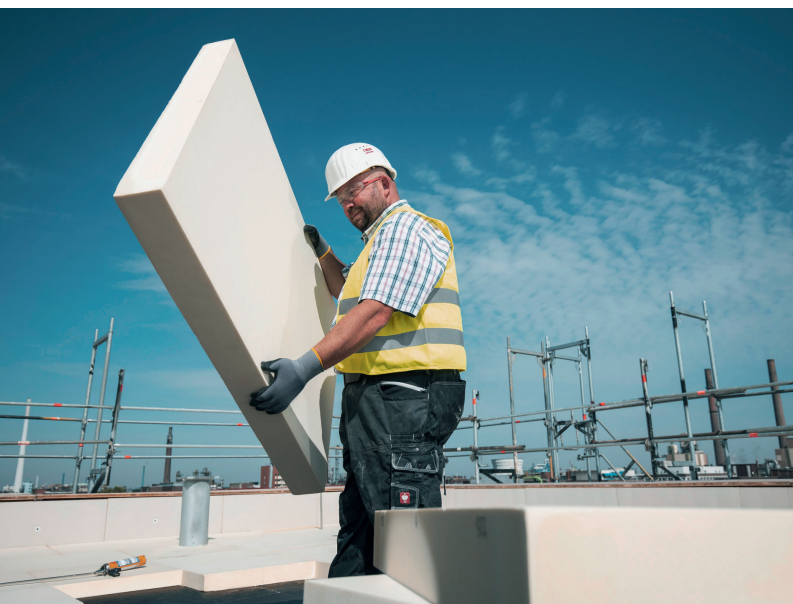
Fig. 2. Climate-neutral MDI can be used, for example, to produce insulating elements made of PUR rigid foam. They provide efficient insulation for buildings. © Covestro
